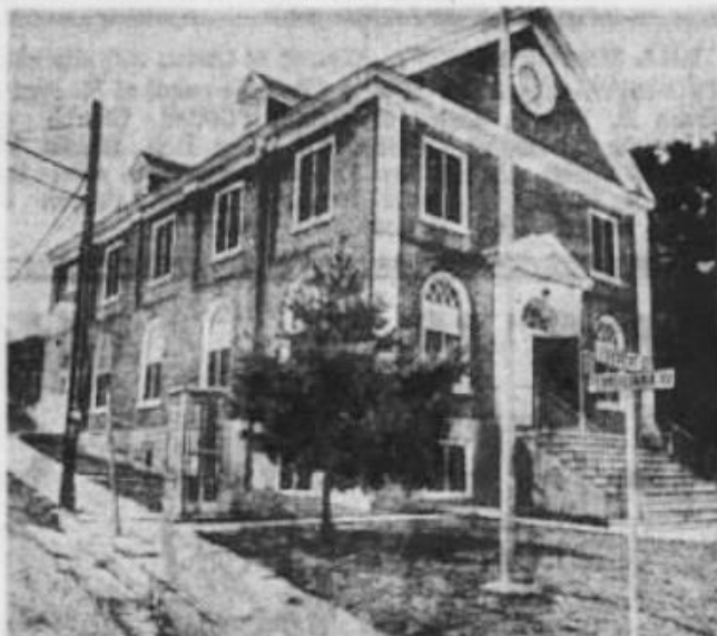
THE COMMUNITY BUILDING houses the public library recently refurbished by the Northeastern Junior Jaycees. Volunteers scraped and scrubbed and painted the dingy, peeling walls to give the library, built in 1920, a bright, fresh look.
